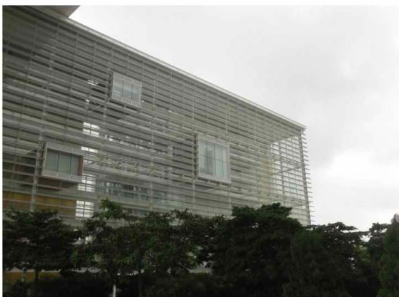
■ KUALA LUMPUR ADMINISTRATION CENTER
